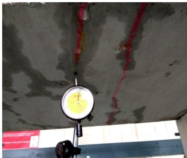
Figure 7 b- Flexural failure at the bottom wythe of slab
